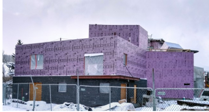
The Pad, a hostel and pub, at Rainbow Dr & Center in Silverthorne built from storage containers.
